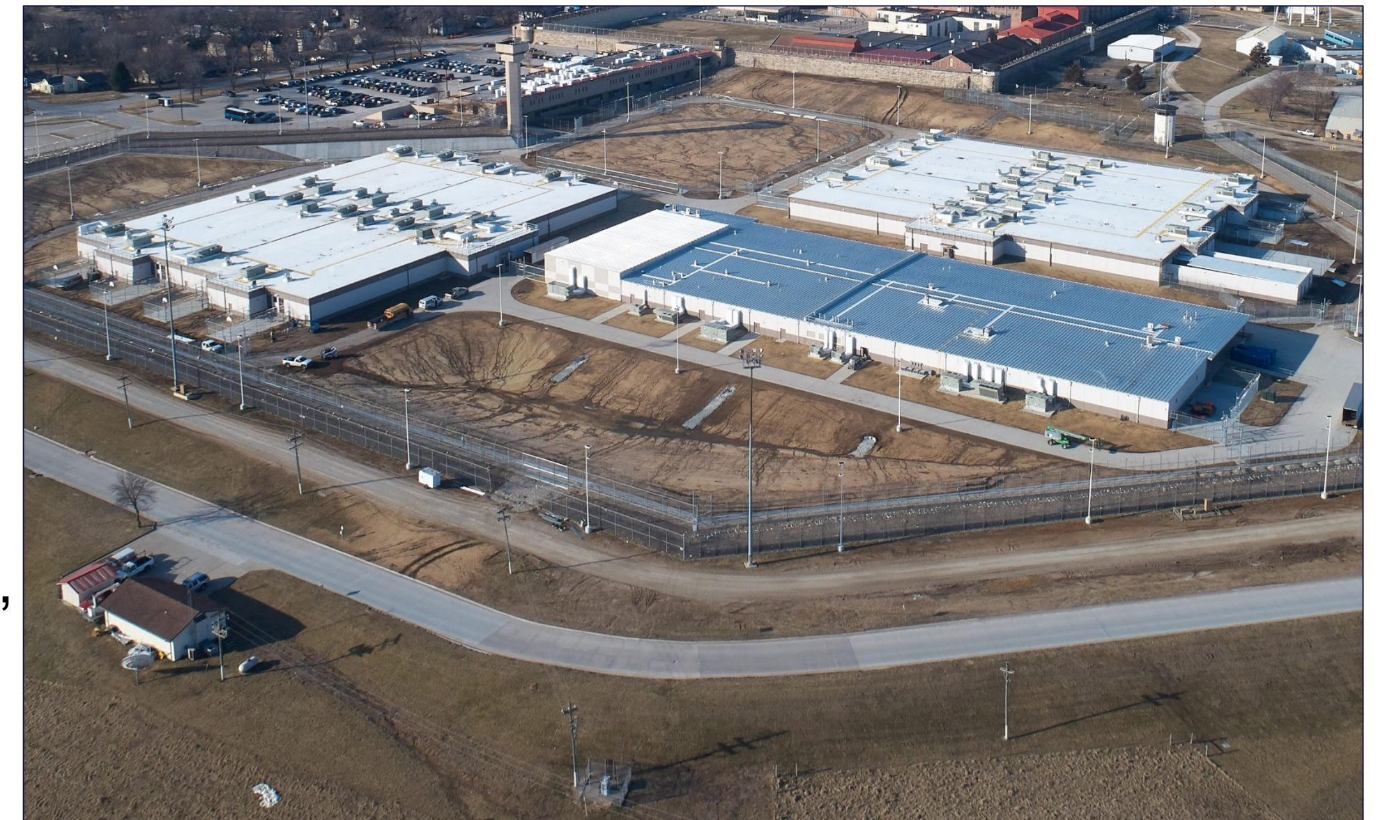
Lansing Correctional Facility, 1,920-bed medium/maximum security complex, opened January 2020
