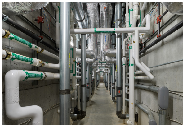
Back mechanical chase providing utilities to all cells, showers, and multipurpose rooms in Housing Units
