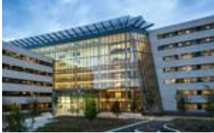
Social Security Administration Office Building in Baltimore, MD acquired by CoreCivic
